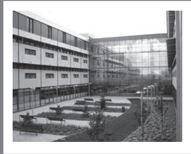
Courtyard at Telford College
